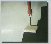
I. Roll and brush one or two base coats of white epoxy depending on surface porosity.
