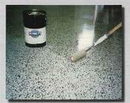
**3.** Remove and collect all excess chips by blowing them and clear seal with epoxy, acrylic, or urethane.
